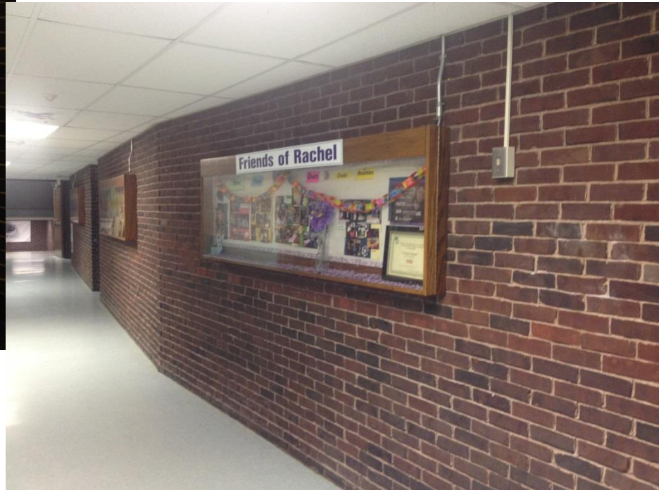
Hallway Next to Auditorium - Fermi
